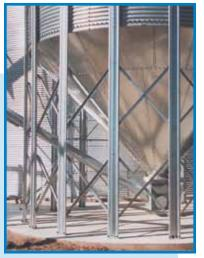
Sturdy "X" bracing between legs gives additional bin strength. Bracing is simple to assemble and offers access to the boot.
