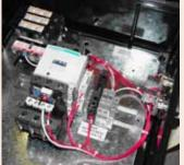
Standard Telemecanique® components are used for safe and reliable motor control.
